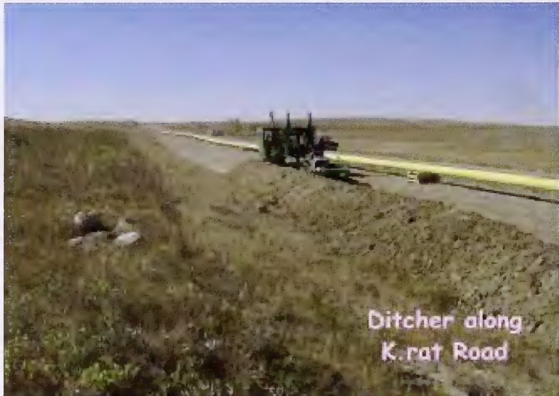
Photo 17 Minimizing disturbance with mid-sized pipe (16 inch pipe)
